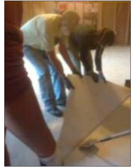
Laurie McCourt from Tallahassee and our Rich Melanson, pulling up flooring
