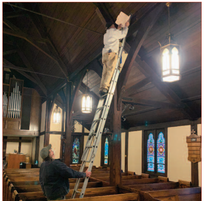
Installing Audio-Visual equipment in the church.
