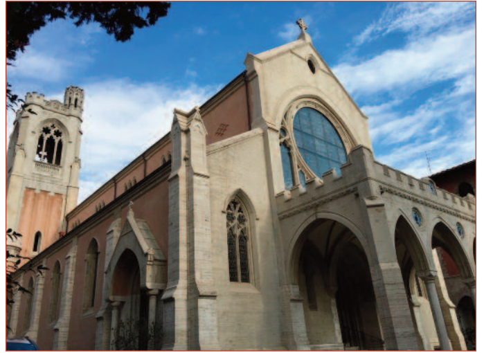
St. James' Episcopal Church in Florence, Italy
