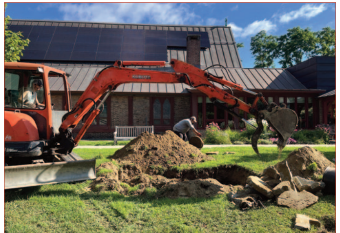
Digging dry well cover broken during roof construction
